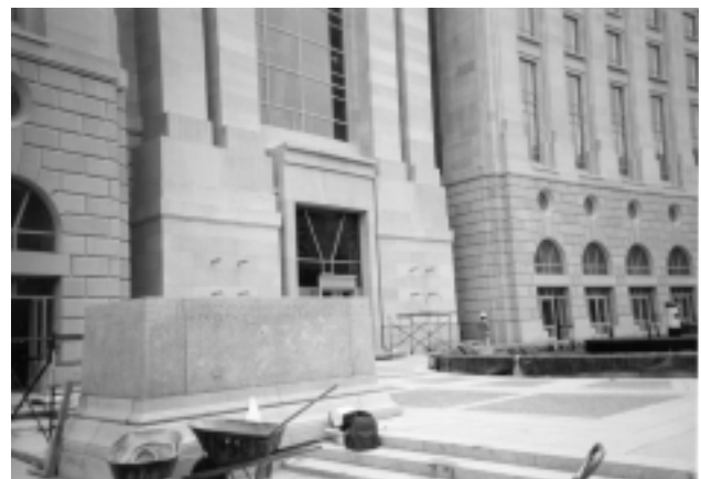
Oscar S. Straus Memorial Construction Site Pedestal on left, Tar paper lined reflecting pool on right
