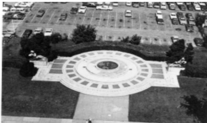
Oscar S. Straus Memorial in the parking lot before reconstruction
