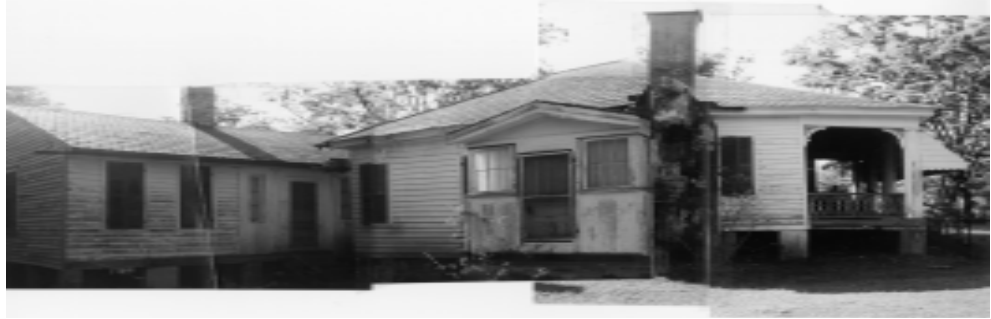
The left side of the house shows an add-on bathroom near the chimney. The el at the rear is the original kitchen, formerly detached from the house. It was later attached with an enclosed porch and walkway.
