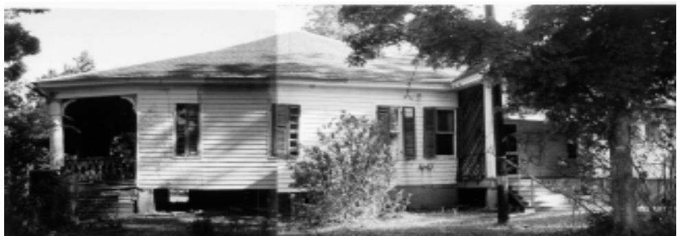
The side porch almost everyone uses these days. It was on these steps that Jean Battle's father was killed by his brother-in-law in 1927, the same day the Strauses went to Atlanta for the opening of the new Davidson Department Store and then visited Talbotton. Mike wrote, "Thank goodness there was no killing in '97; maybe we've changed our luck."
