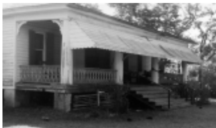
The front porch with "Sheaf of Wheat" pattern railing which is very common on a house of this age in Talbot County.
